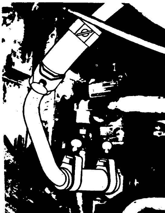
FIGURE 3-9. Satisfactory oil line installation.
